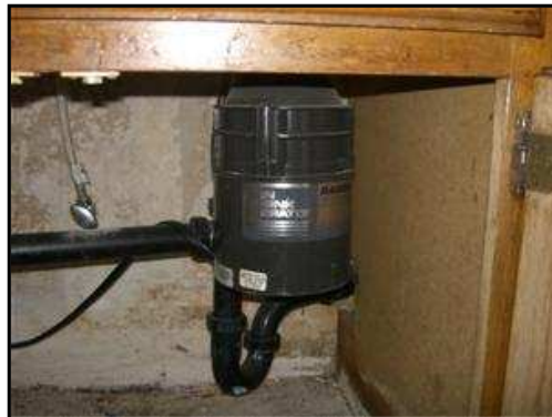
6.12.A Picture 1 Food waste disposer non-operational.
