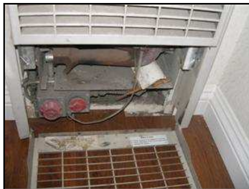
6.14.A Picture 1 Debris present near burner.
