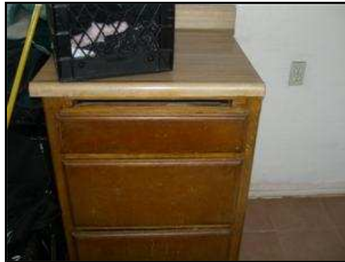
6.5.A Picture 2 Breadboard missing.
