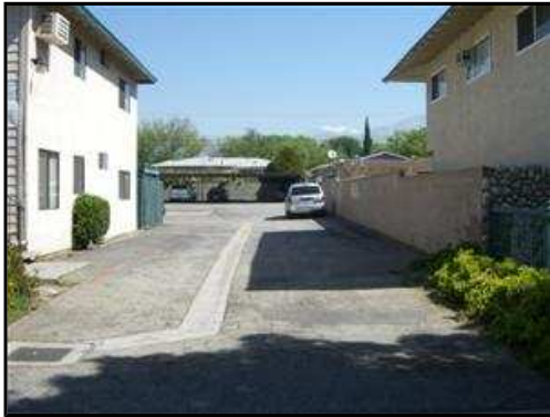
2.8 Picture 1 Asphalt driveway
