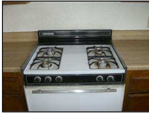
6.10.A Picture 1 Burners functional, igniter non-operational.
