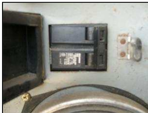
7.1 Picture 4 (1) 100 amp disconnect per meter.
