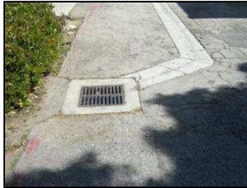
2.8 Picture 2 Appropriate swale and run off drain present.
