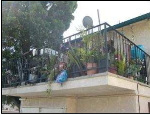
2.3 Picture 5 Excessive storage on balcony.
