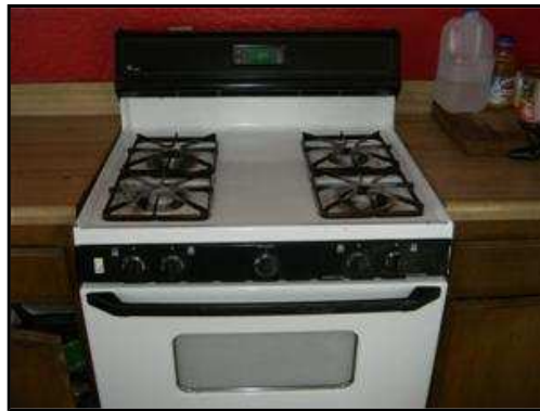
6.10.B Picture 1 Burners functional - igniters non-operational.
