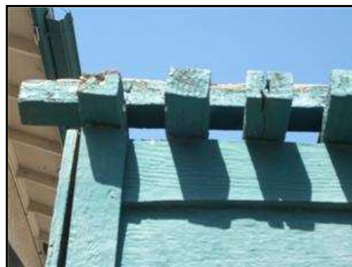
2.3 Picture 4 Trash container overhead cover.
