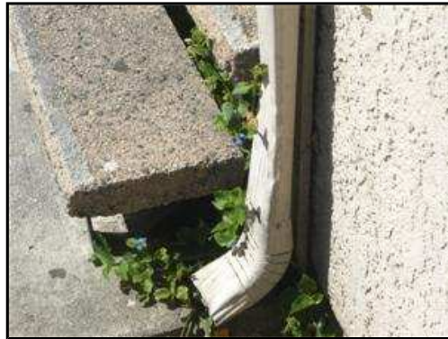
1.4 Picture 1 Rain gutter downspout damaged.
