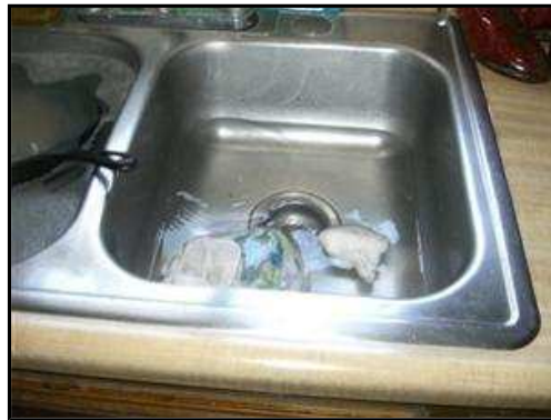
6.5.E Picture 2 Slow kitchen sink drain.
